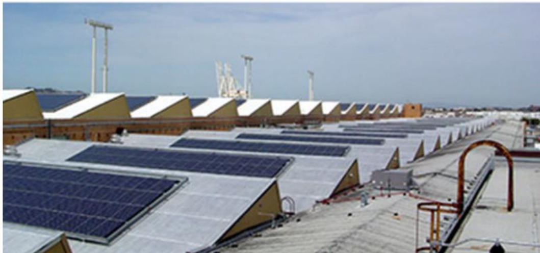
Figure 23. Solar collectors installed in a compatible manner on low sloping sawtooth monitors. Top Photo: Neil Mishalov, Berkeley, CA.
