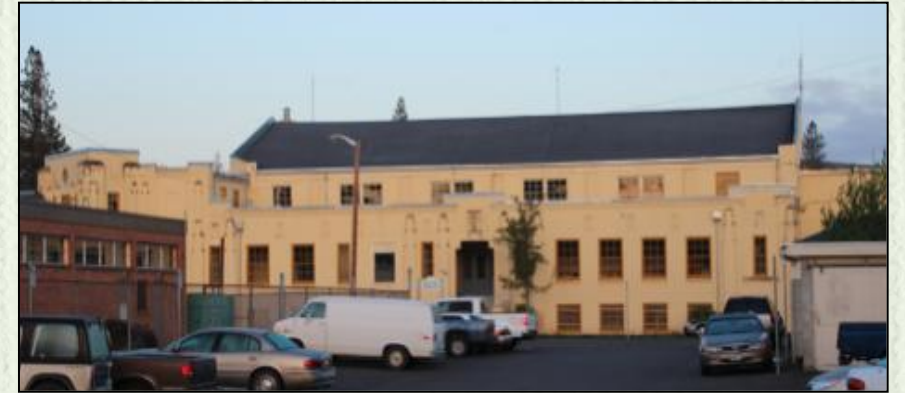
Armory Window Repair – Cottage Grove
